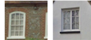
Decorative brickwork detailing, quoins/ dressings | Light painted render
