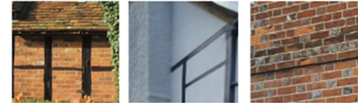
Timber frame with brick infill | Painted peddledash and render | Handmade facing brickwork - red / orange with grey/ blue/ burnt
