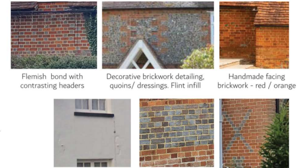
Flemish bond with contrasting headers Decorative brickwork detailing, quoins/ dressings. Flint infill Handmade facing brickwork - red / orange Painted render English bond Contrasting brickwork bands Decorative brickwork
