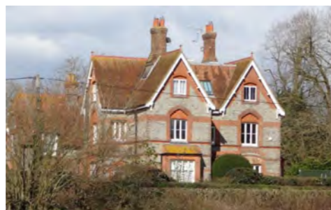
The former Vicarage - now Glebe House - Locally important building
