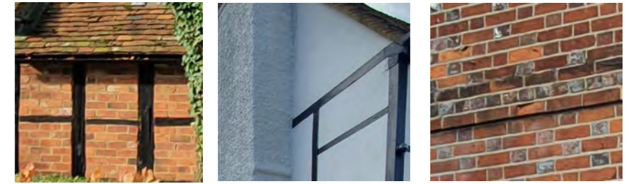
Timber frame with brick infill
