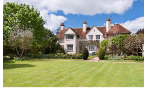
Eyot House - Grade II* Listed
