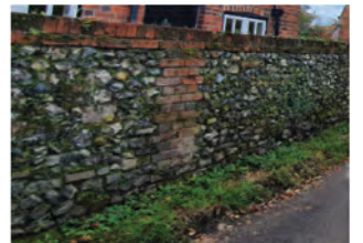
Walled front boundary - brick or brick/ flint - red orange
