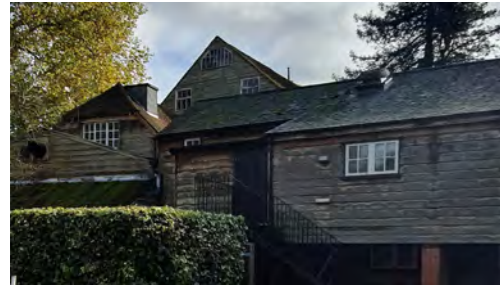
Sonning Mill - Grade II Listed
