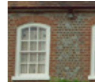
Decorative brickwork detailing, quoins/ dressings
