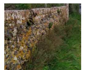
Walled front boundary - brick or brick/ flint - red orange
