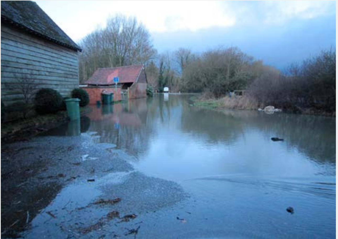
■ Old B478 Flooding, 2009
