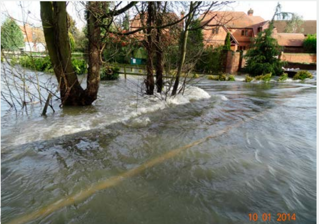
■ Flooding of the B478: the road acts as a dam until it is topped
