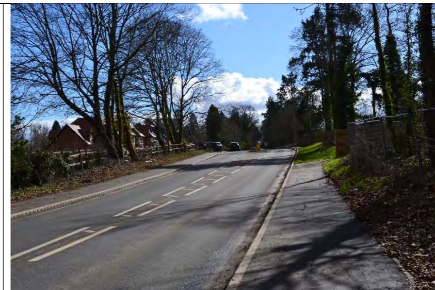
View southeast along the A4155, Reading Road, on the eastern boundary of the PLCA
